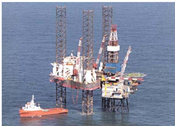
© Wintershall Q4-C platform, North Sea
